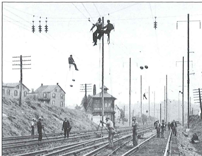
Linemen putting the final touches on a multi-track catenary system by working from the supporting messenger. They are installing sectionalizing insulators, adjusting hanger brackets, adjusting messenger tensions and other final tasks.
