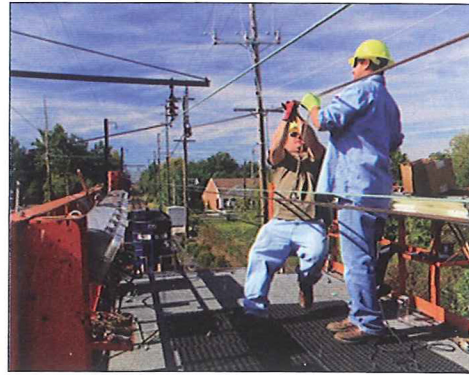
Southeastern Pennsylvania Transportation Authority linemen working on their overhead catenary from a wire train. (Photo Courtesy SEPTA)
