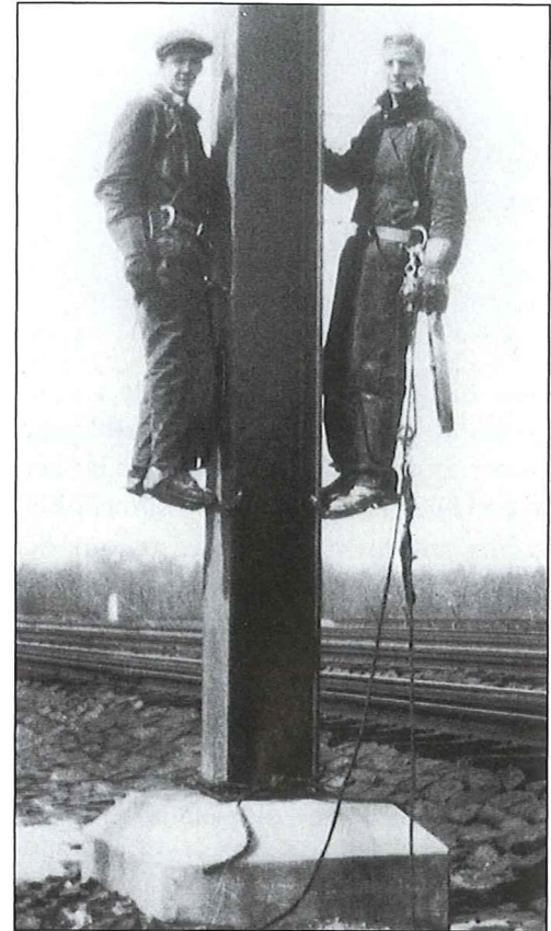
William Wister Haines (R) and a fellow lineman on a catenary structure wearing the special climbers called "skates" that were utilized for climbing catenary supporting steel structures.
